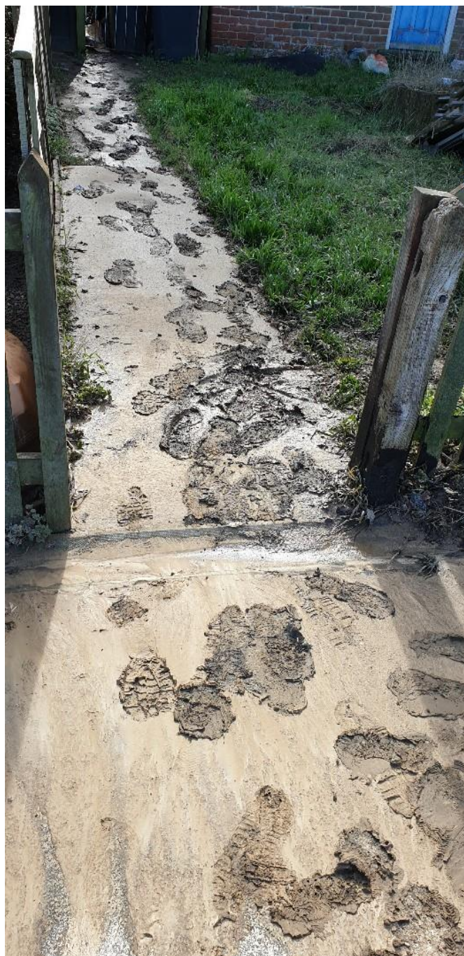
Mud over flow in Thanington Road caused when mud was able to flow from new development in the drain system in Cockerling Road. Photo by Cllr Toni Baker.
