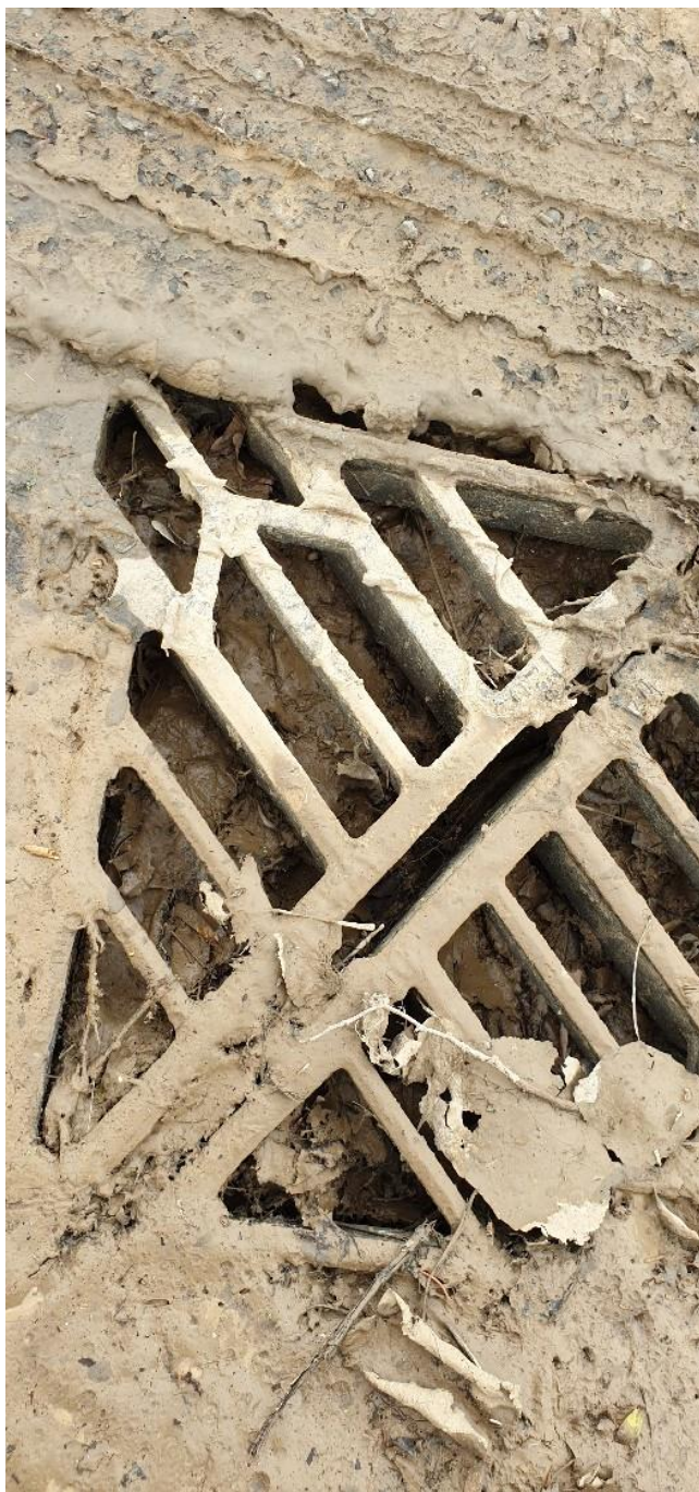
Mud over flow in Thanington Road caused when mud was able to flow from new development in the drain system in Cockerling Road. Photo by Cllr Toni Baker.
