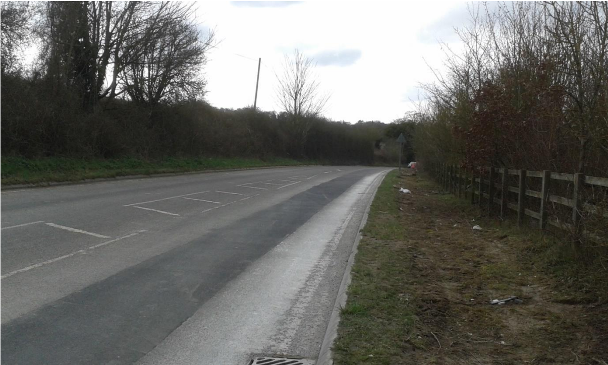
3/ View of the approach on MILTON MANOR ROAD to the COCKERING ROAD junction looking towards the CHARTHAM direction, showing the blind brow and road curve
